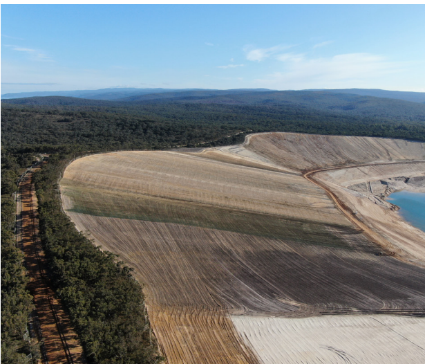
An aerial of the mine's south wall showing the progress of the hydroseeding program. Coalmine Rd is shown on the left.
