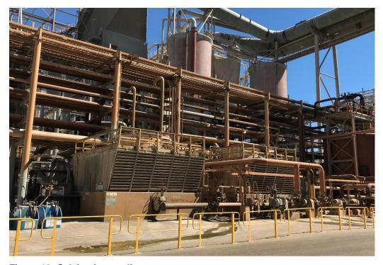
Figure 19: Calcination cooling towers
