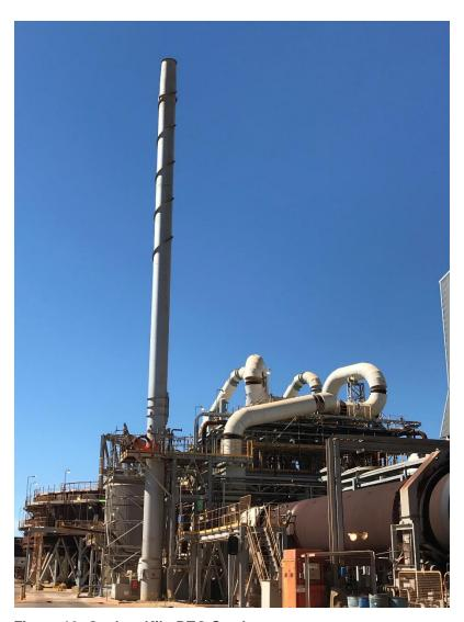
Figure 10: Oxalate Kiln RTO Stack
